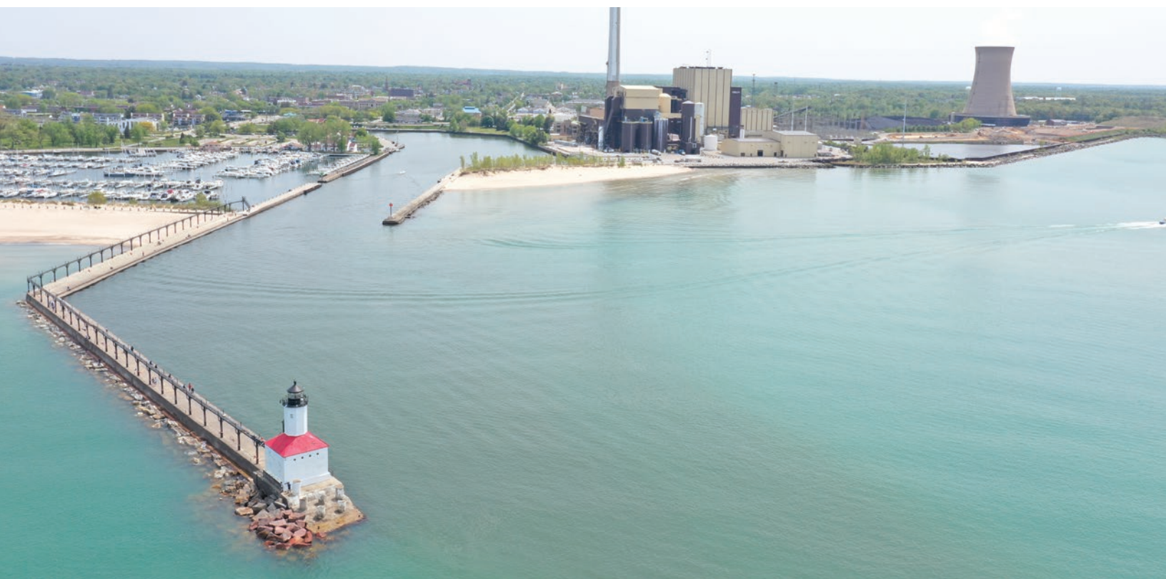
Photo: Michigan City Harbor | Michigan City, Indiana, courtesy of Anderson + Bohlander
