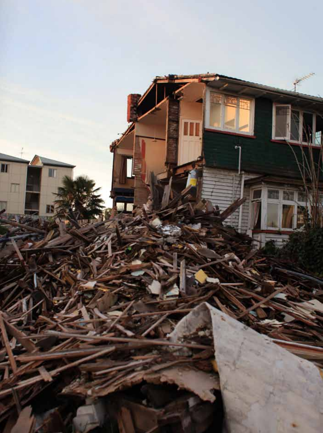
Earthquake damage, Christchurch, New Zealand. Photo: © Alexandra1977 | Dreamstime.com
